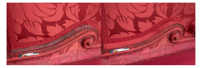
Figure 6. Area of silk loss before treatment (left) and after the papier-mâché dust protection was applied (right) ©Royal Collection Trust/© H.M Queen Elizabeth II
