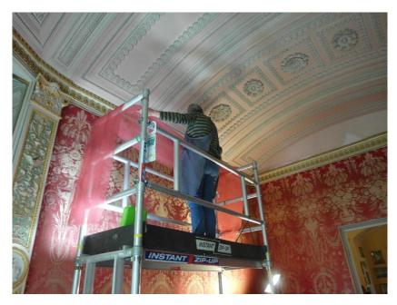
Figure 10. Installing a final layer of protective conservation net, dyed to match the pink silk. © Ksynia Marko
