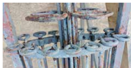
Above: The outer frames all contained a distinctive and unusual fire weld
