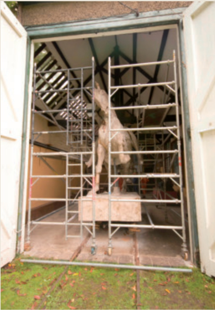
Scaffold up around Physical Energy
