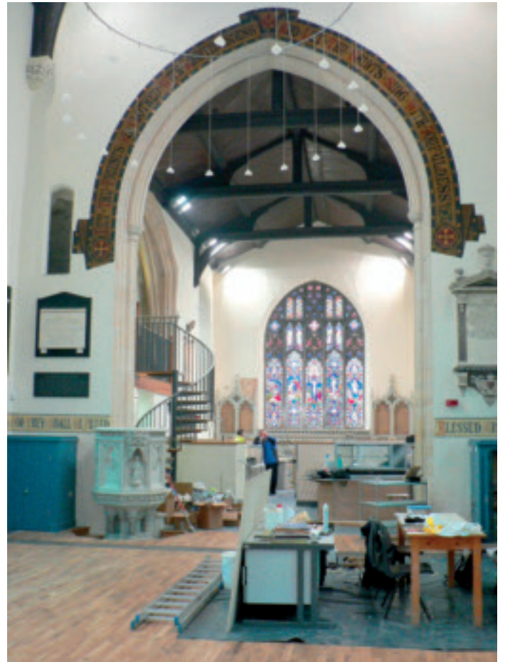
The interior ready to be transformed into a café
