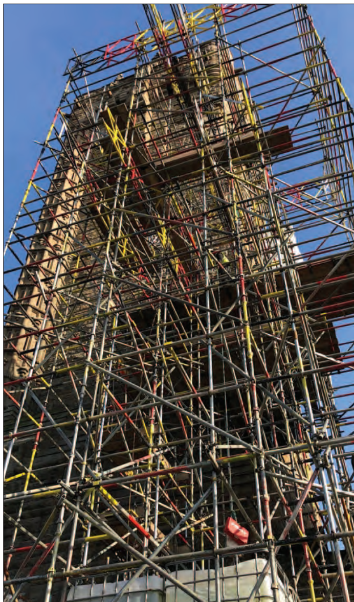
Scaffolding with twenty tonnes of counterweights and lifting beam
