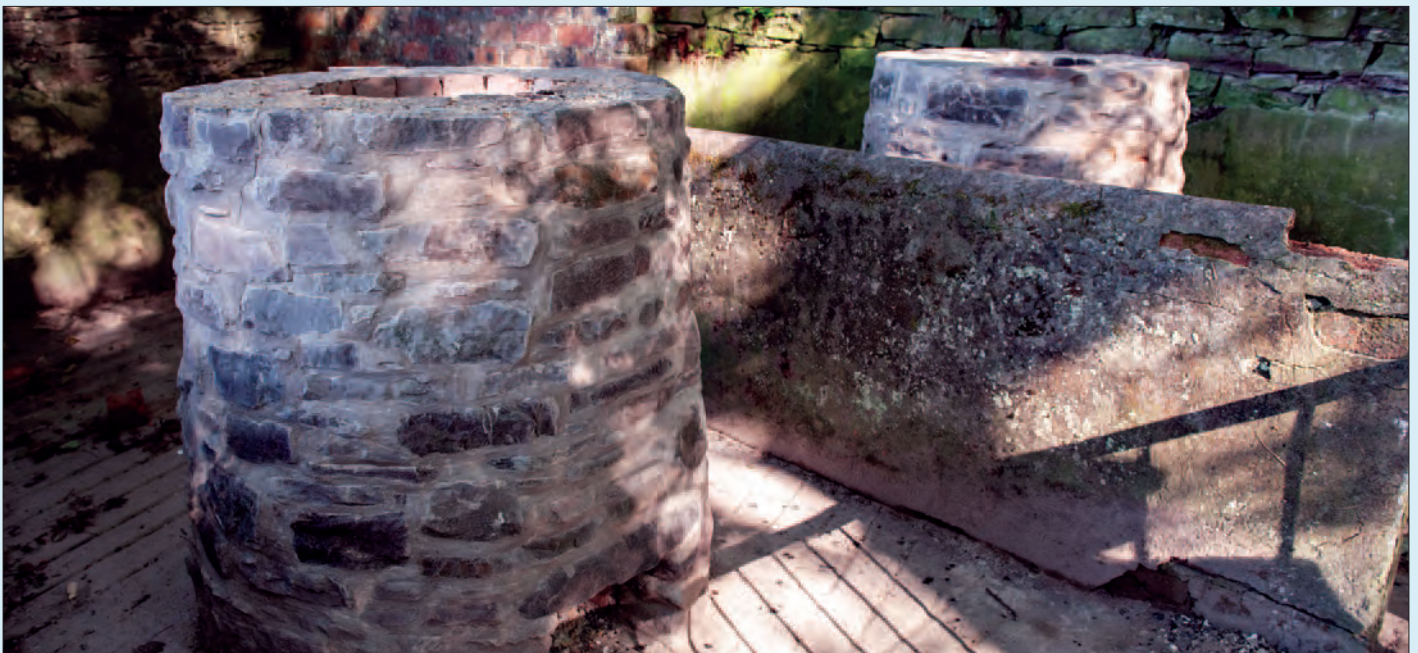
Kiln for small-scale lime burning at Charlestown
