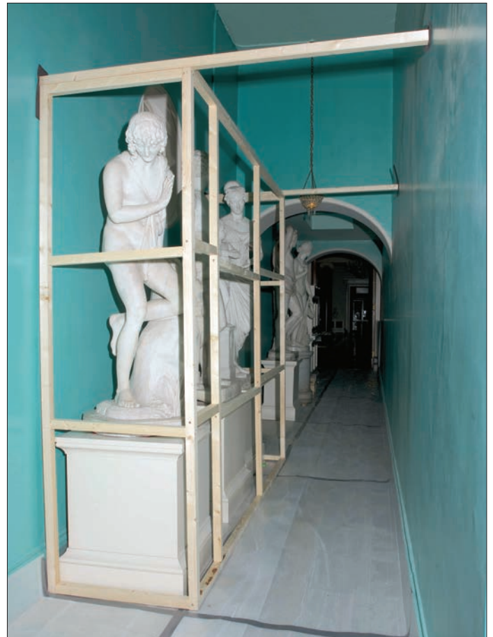
Removing the sculpture to the adjacent east passage, which had been load tested, and protected in situ
