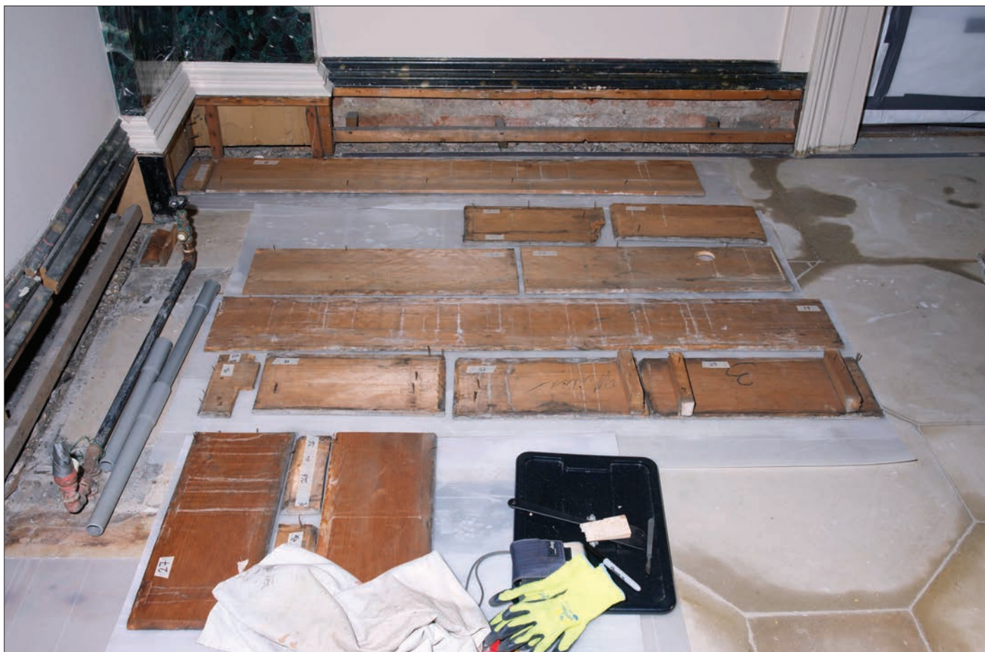
The skirting boards were removed with the help of a furniture conservator, labelled, and documented before being conserved on site
