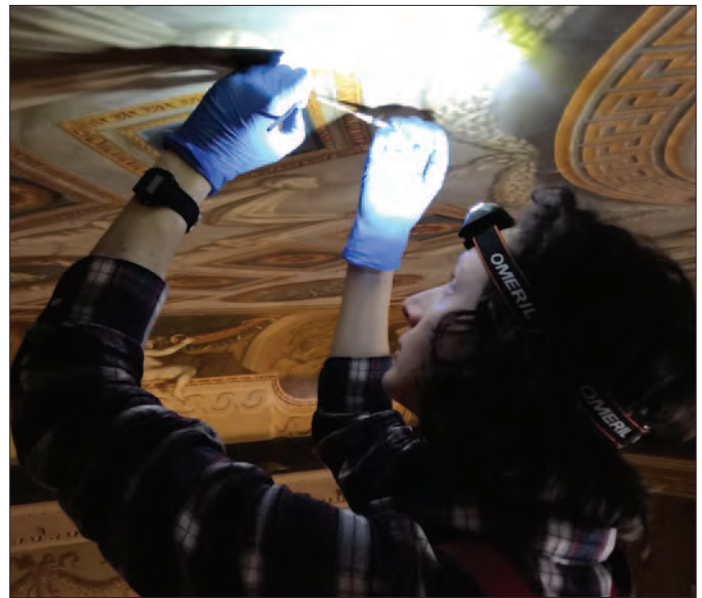
Flake fixing at Hampton Court Palace: the project was literally a highlight for Elizabeth Woolley ACR in headtorch and on a cherry-picker
