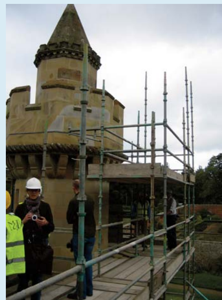
Looking closely at the external work
