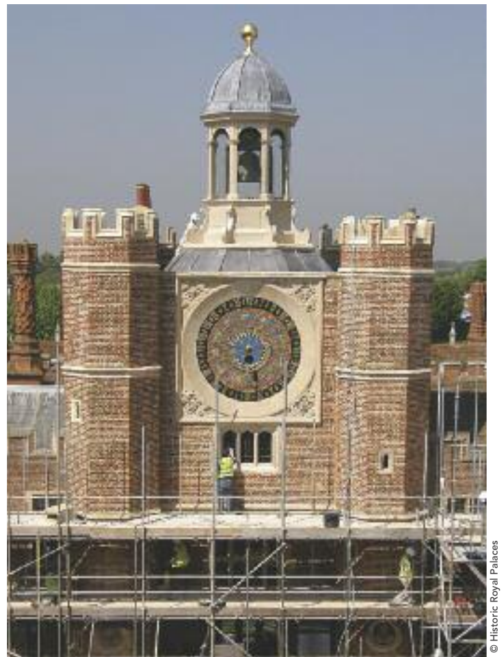
Figure 12: As work nears completion on the Anne Boleyn Gatehouse the restored cupola and clock are revealed – May 2008.
