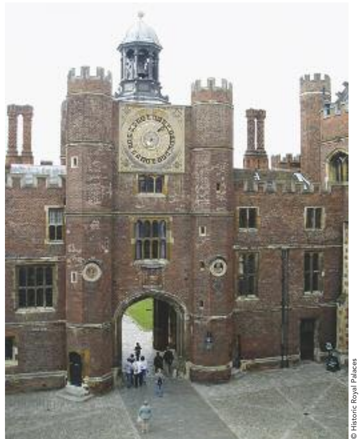
Figure 1 The Anne Boleyn Gatehouse, Hampton Court Palace before building conservation work. The clock sits 15 metres from ground level.
