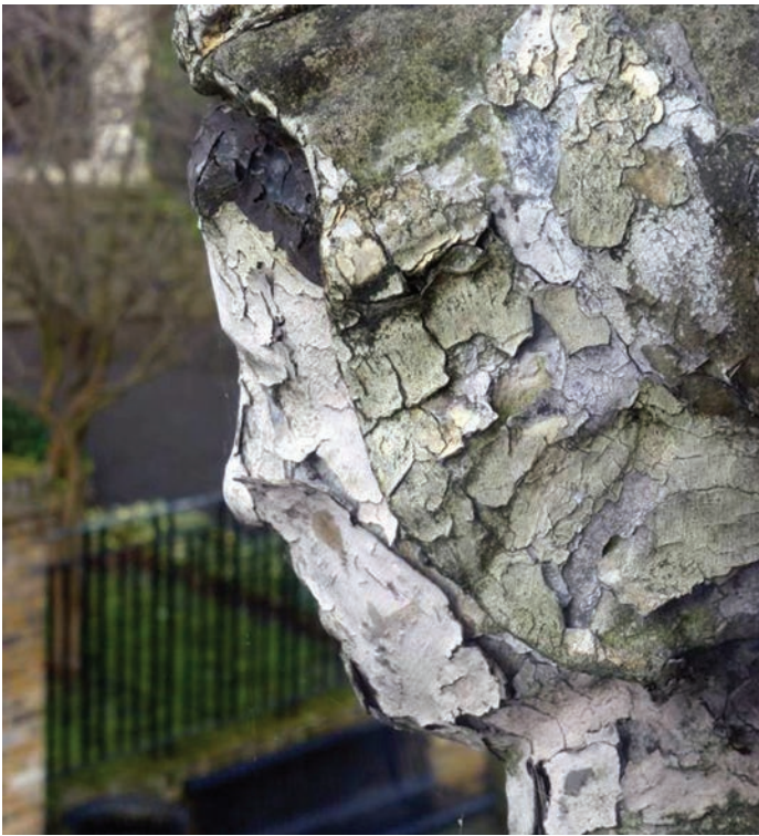
The girl's face showing layers of paint peeling off
