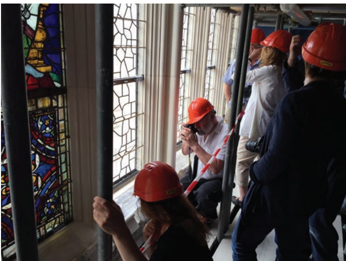
Stained Glass Group members view the reinstallation of the Great South Window at Canterbury Cathedral
