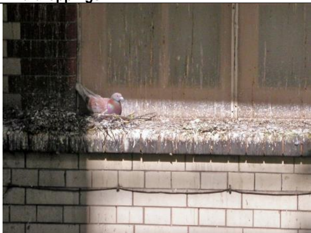
A windowsill with a large build of droppings from a nest site.
