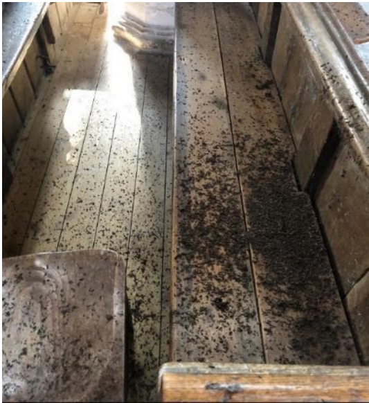
A large accumulation of droppings beneath a roost entry on a church pew
