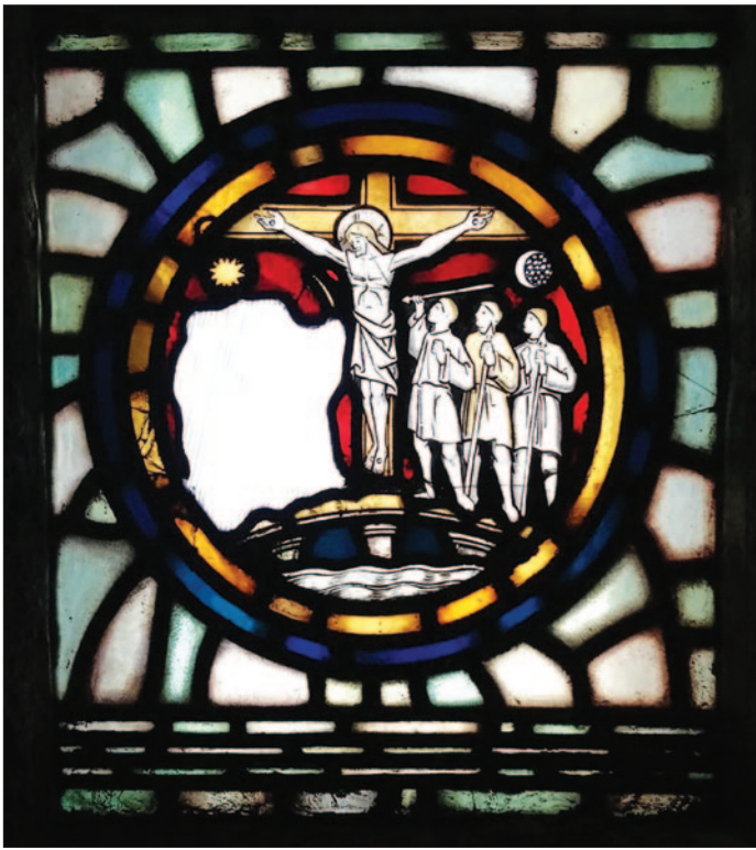
The damaged embrasure window with the broken piece removed in situ. The replacement piece is shown below
