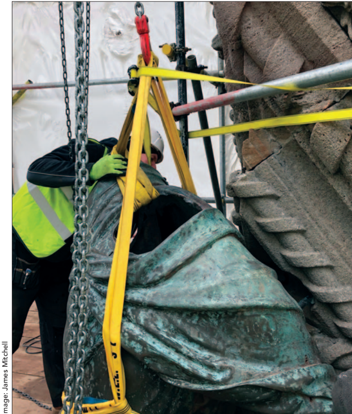
This shows the torso released and ready to lift. The proximity to the stone niche can be seen
