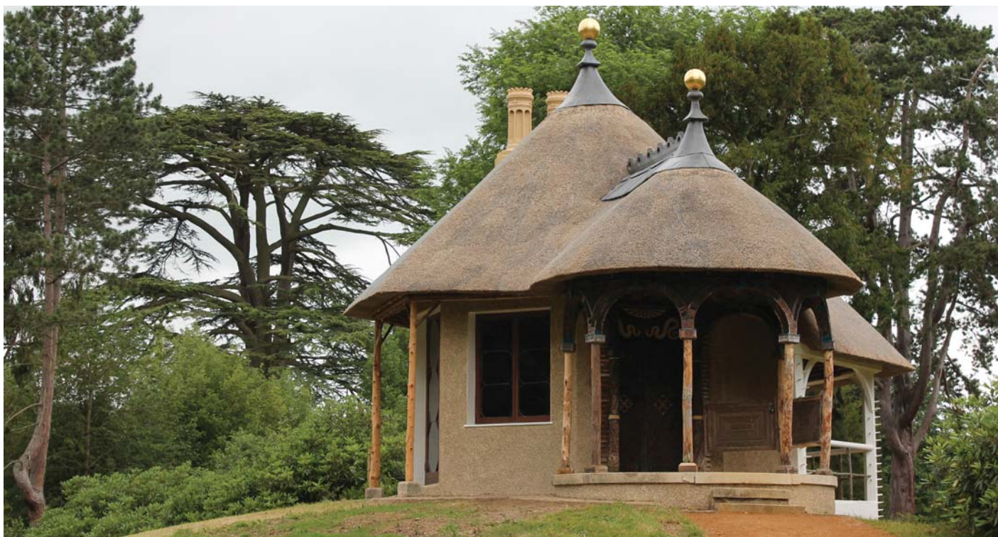
The completed Cottage
