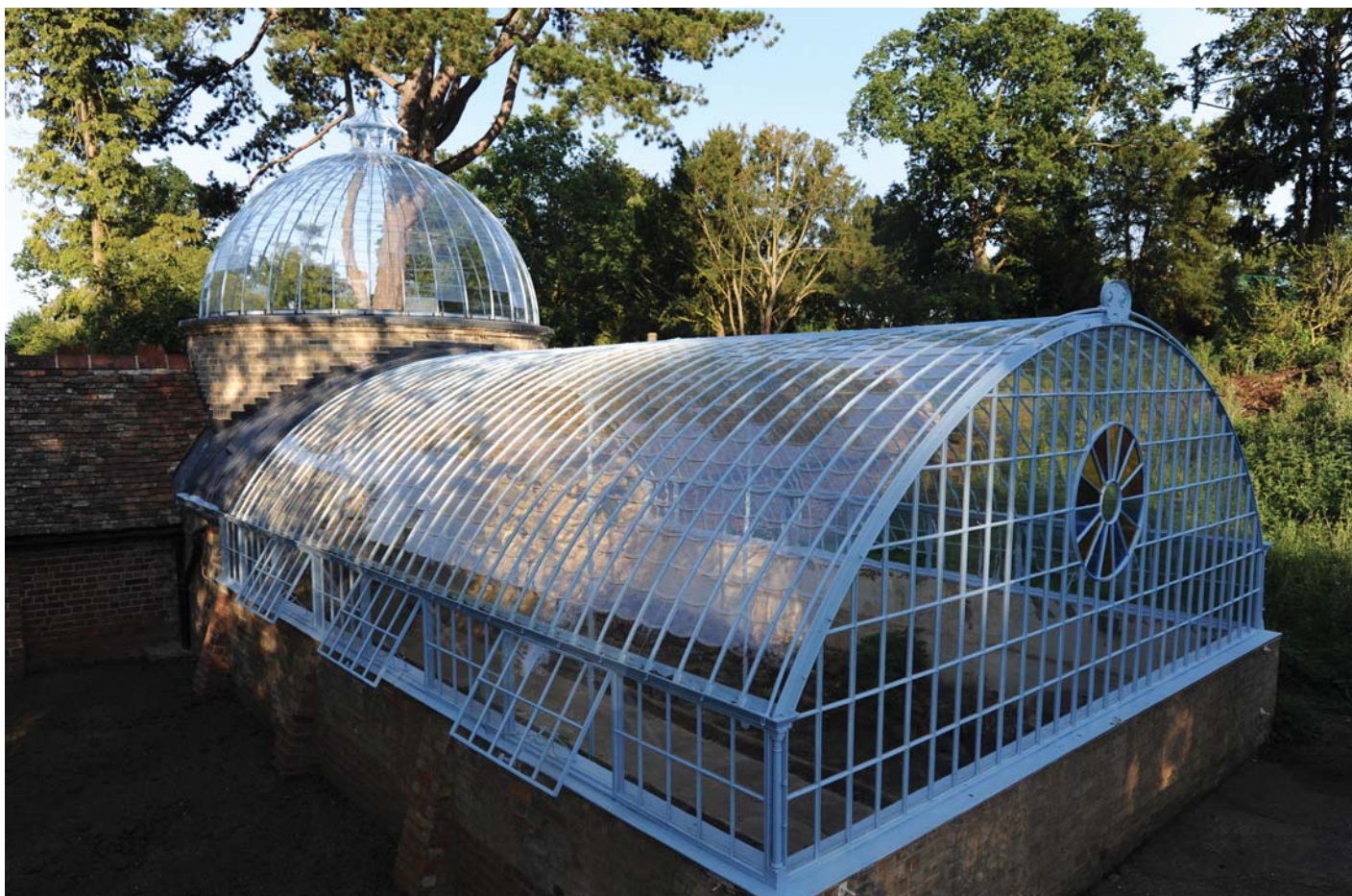
The restored grotto-ferney in its finery
