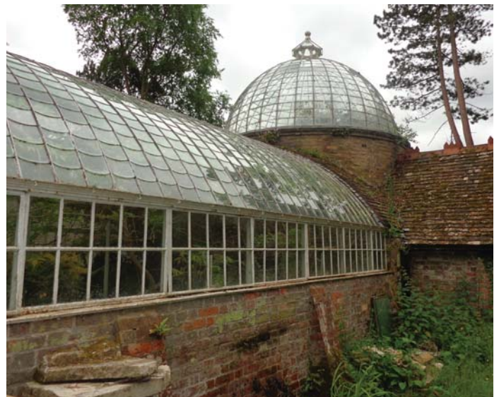
The grotto-fernery prior to works
