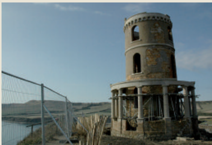
Clavell Tower as it stands on a crumbling cliff face
