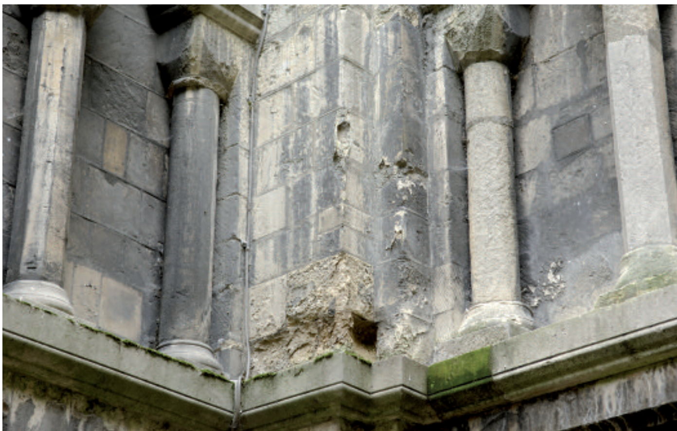
Decaying stonework on the North side of the Cathedral
