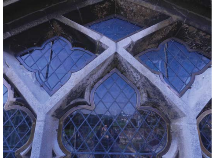
Above: detail of tracery sections formed using water jet technology
