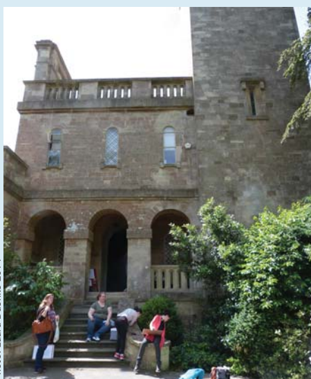
Building surveying at Beckford's Tower
