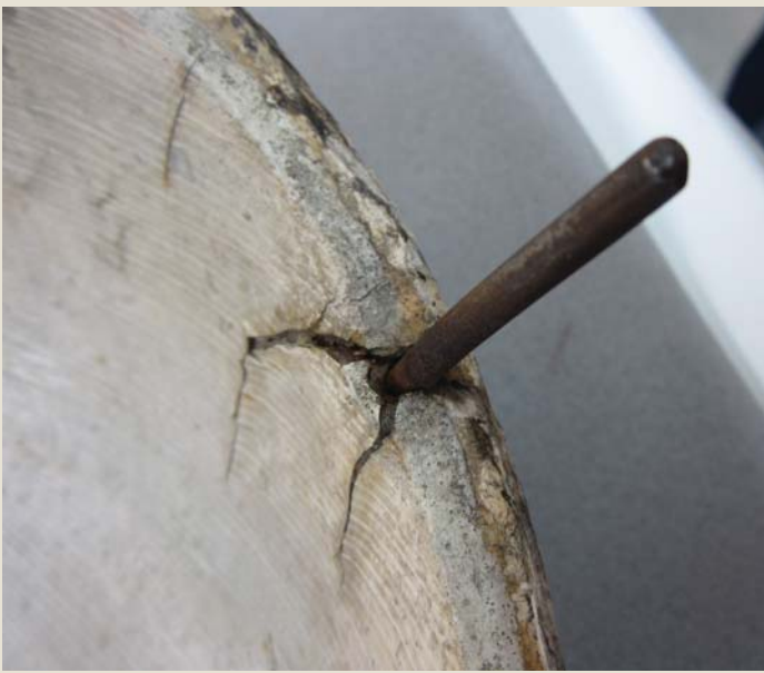
Shell before treatment showing corroded metal, lifting paint
