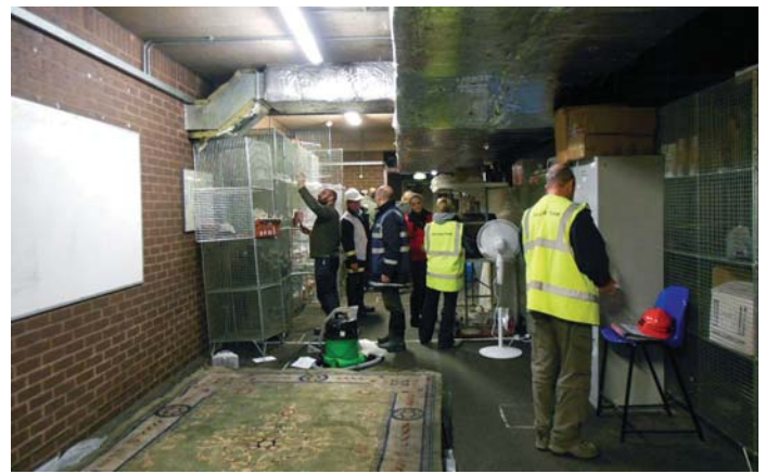
Inside the wet recovery area
