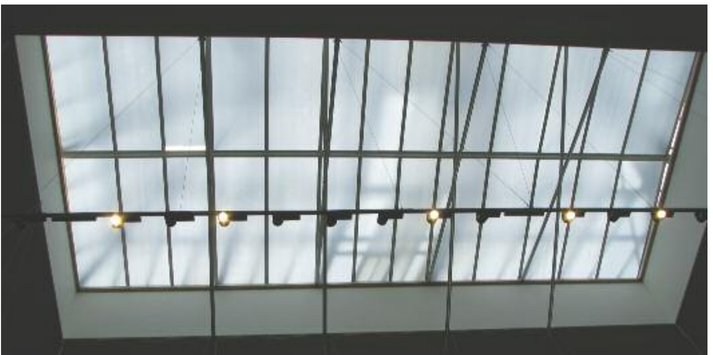
New laylights with new filter and LED lighting
