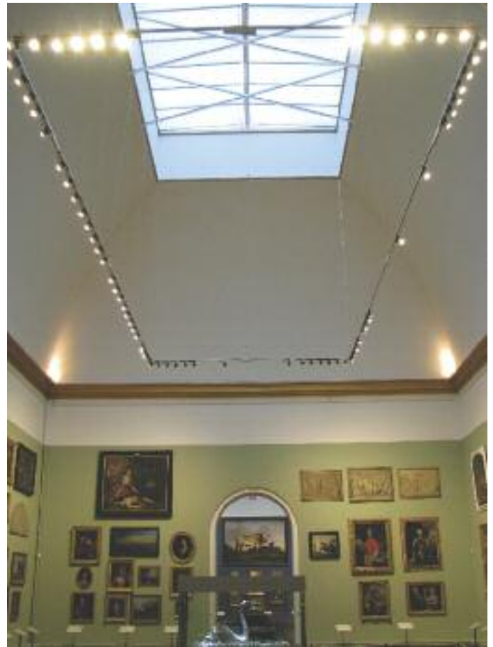
New laylights with new filter and LED lighting
