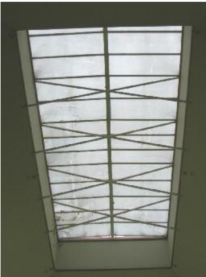
Laylight with old glazing and filter
