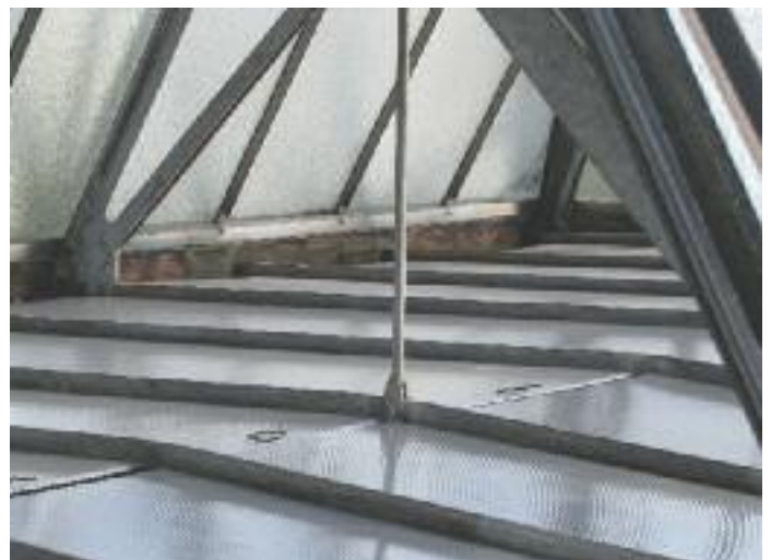
The new system. Twin wall with film attached in atrium space
