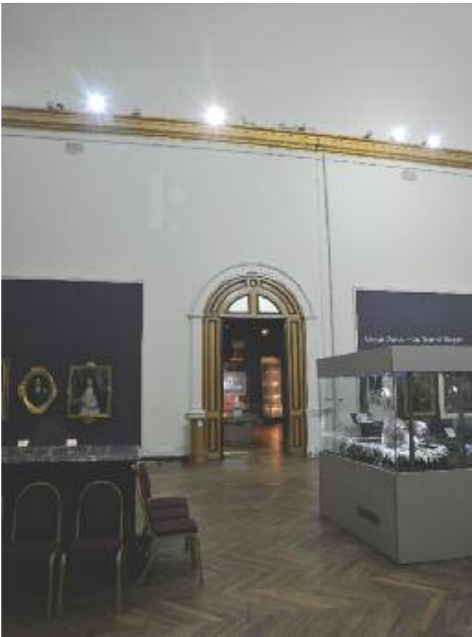
The old lighting system in the Centre Picture Gallery
