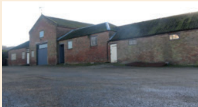
View of the North façade of the suite of new studios, before building works completed.
