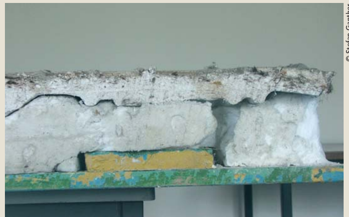
In cross-section, the ceiling rests on foam
