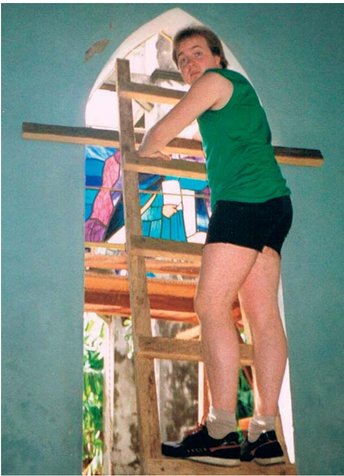
Fitting Paul Quail windows in Nigeria 1991
