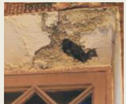
Water ingress has damaged the plaster
