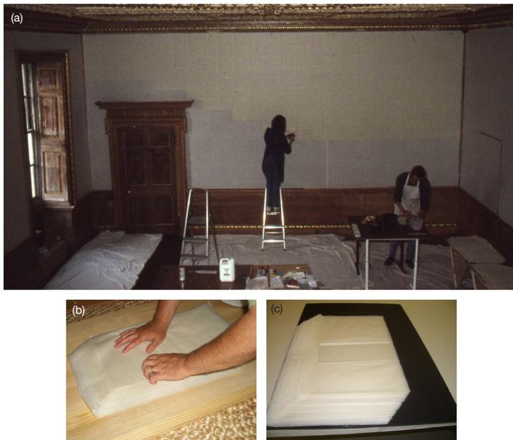
**Fig. 15** (a) Wall preparation incorporating a floating layer, *ukekake*. (b) small sheets of knife- and water-cut paper; (c) paper sheets stacked and ready for pasting. Photograph reproduced courtesy of Mark Sandiford of Sandiford & Mapes.
