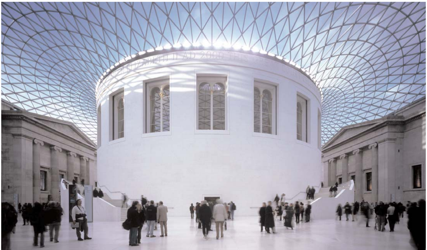
British Museum: looking north from the South Portico into the Great Court. Many new museum buildings of recent years incorporate a great deal of glass, which can cause overheating. The roof of the Great Court includes natural ventilation designed to maintain moderate temperatures.
