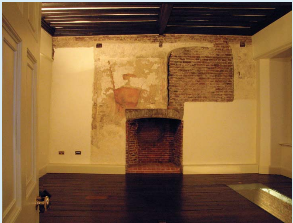
Bromley by Bow. The south wall of the boardroom conserved with all historic sequences presented. A Tudor window was found bricked up just after 1710 when the room was panelled, and the fireplace and sash windows were inserted. In the centre of the picture, the fragmentary remains of at least three historic paint schemes dating from the 16th to late 17c have been conserved by Andrea Kirkham. The earliest of these sequences, a male bonneted figure holding a longbow, pennant or staff dates to the second quarter of the 16c. The remainder of the room is presented as early 18c, minus the panelling which was removed in 1952. (Note and image courtesy of Paul Latham)
