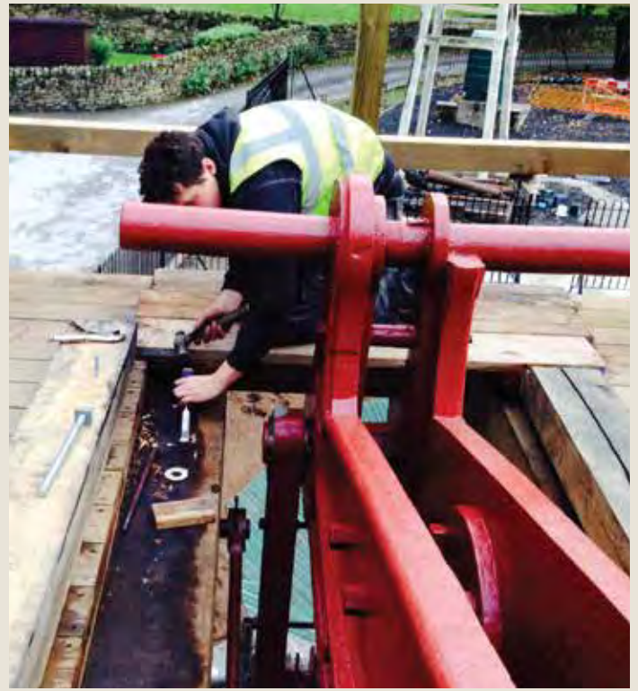
An intern sponsored by Historic Scotland works on the new timber
