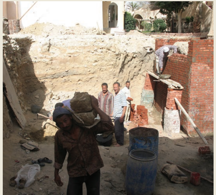
Building work starts
