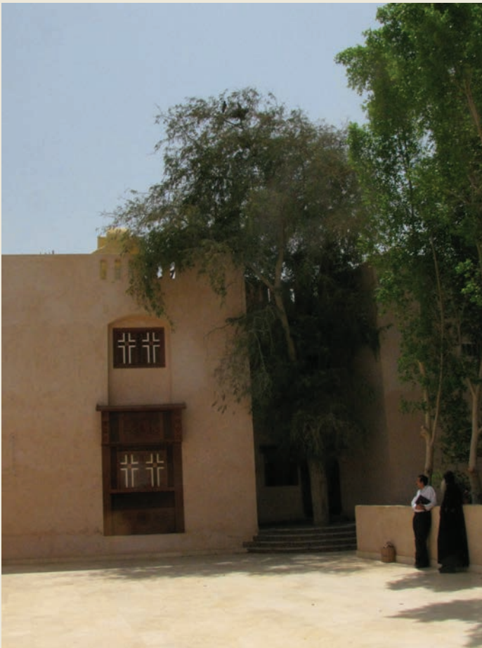
The East side of the building completed in 2012
