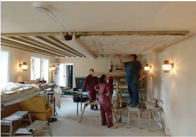
The trainees under direction as the ceiling is reinstated
