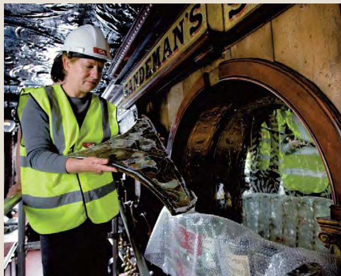
Mosaic glass panels above the bar – removal from the fascia
