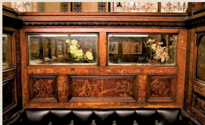
Reverse print mirrors in the snugs – damages and graffiti
