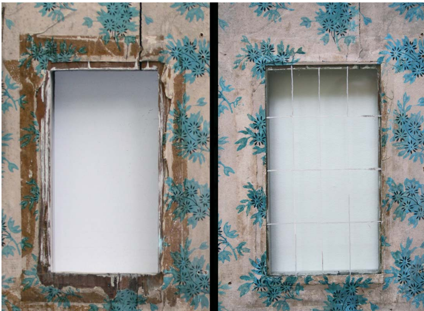
The window surrounds before and after conservation
