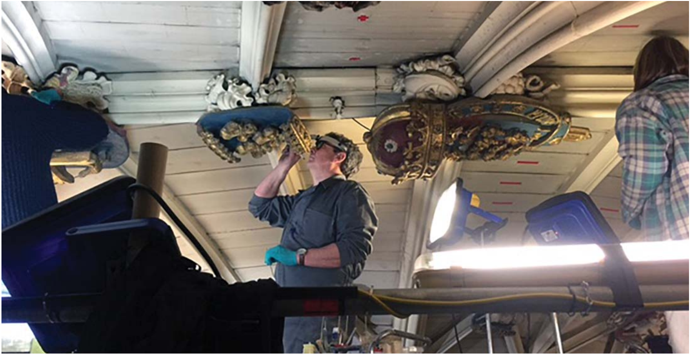
Working on the ceiling bosses in Winchester Cathedral
