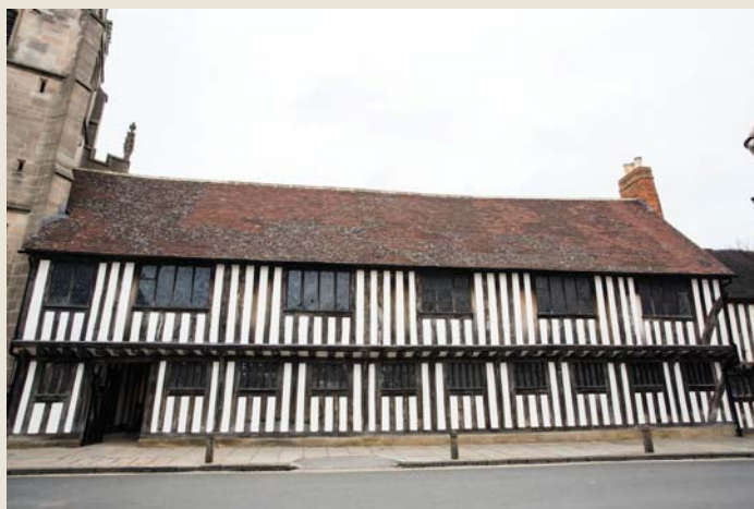
The exterior of the Guildhall and schoolroom
