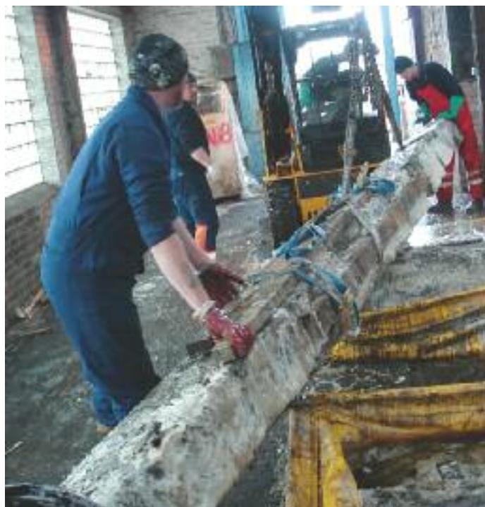
Contractors removing timbers from treatment tanks
