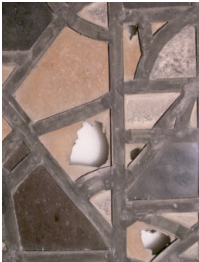
Fig. 5 CHnIX panel 8a reflected light showing corrosion damage and breaks
