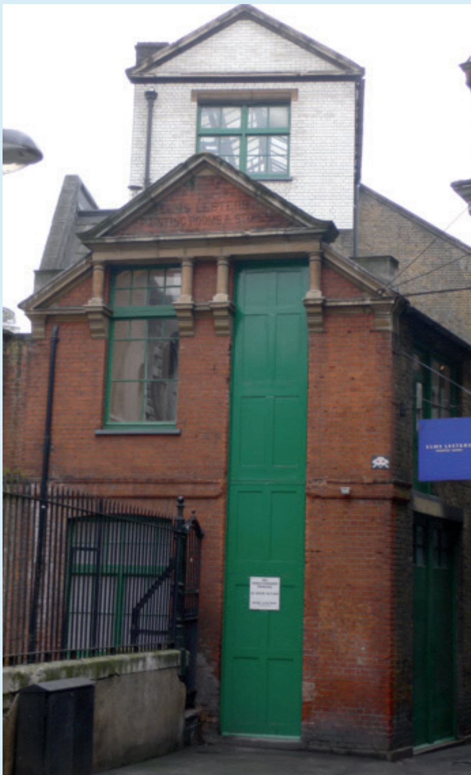
Elms Lester Paint Frame
