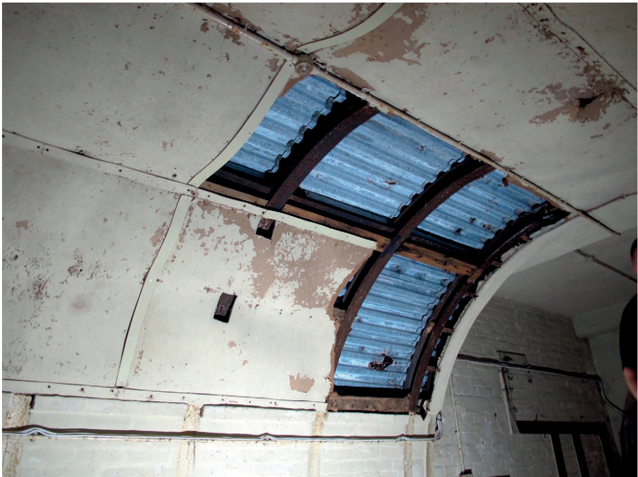
Figure 4 Removal of non-historic, wood borer-infested lining panels from the tunnels (© English Heritage 2021).
