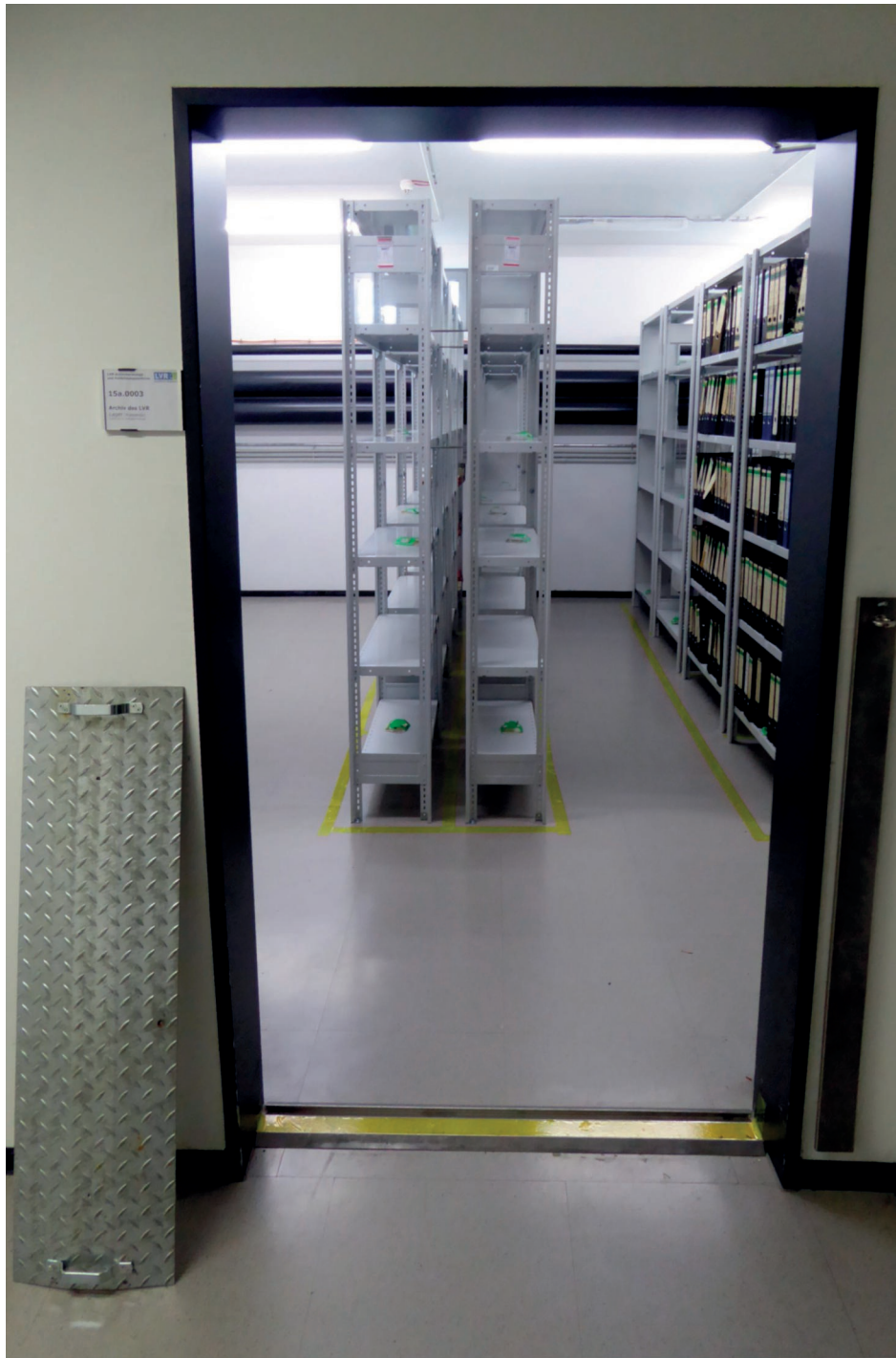
Figure 3 View into the quarantine room. The M-style barrier is fixed permanently to the floor on the threshold with the yellow adhesive tape inside the barrier. Quarantine racks are surrounded by the double-sided adhesive tape (© Volker Hingst 2021).
