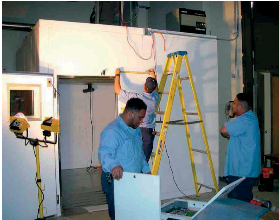
Figure 2 Installation of the blast freezer at the Ransom Center in 2003 (© 2021 Alan P. Van Dyke).
