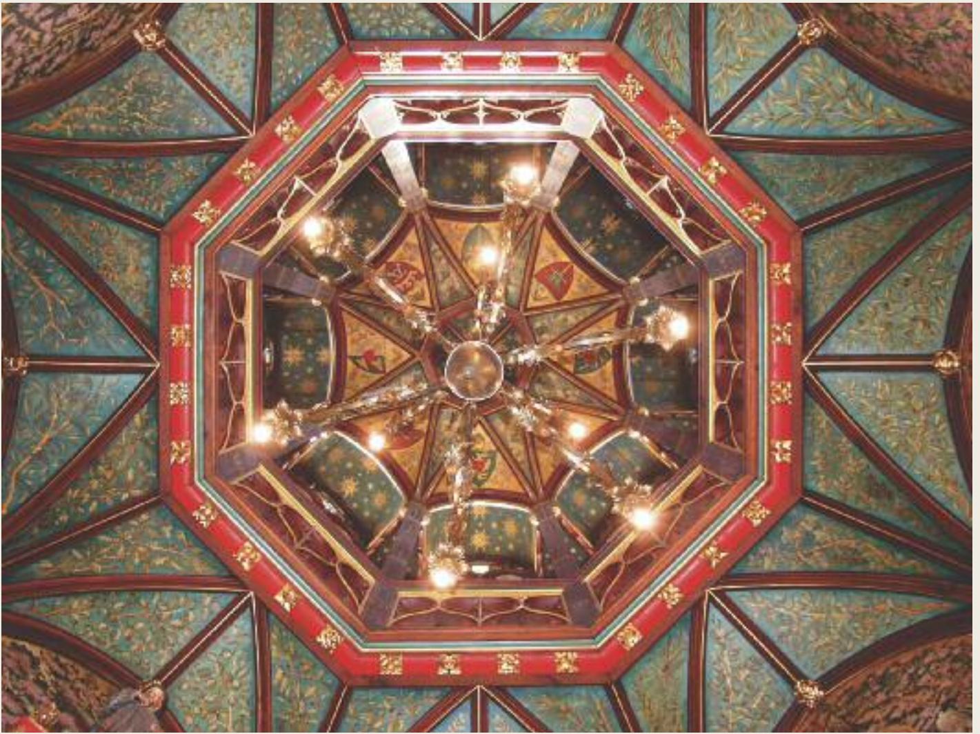
Chaucer Room ceiling
