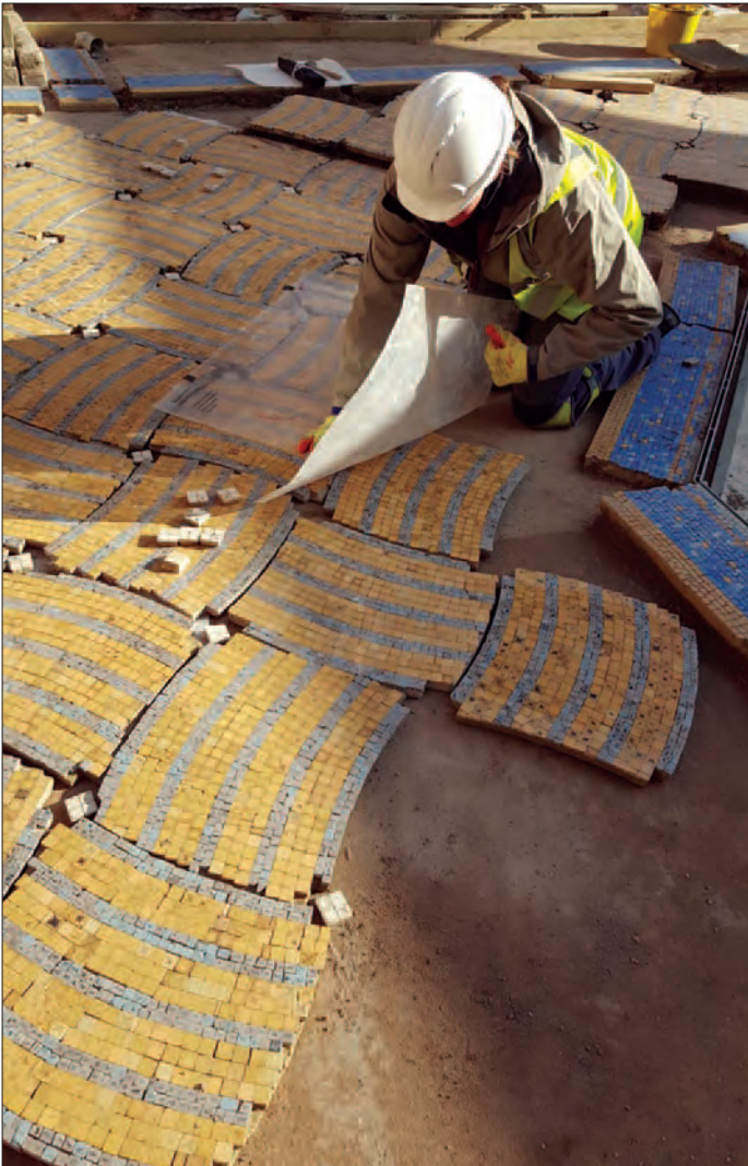
Laying the floor panels out dry and checking their alignment with an acetate of the design
