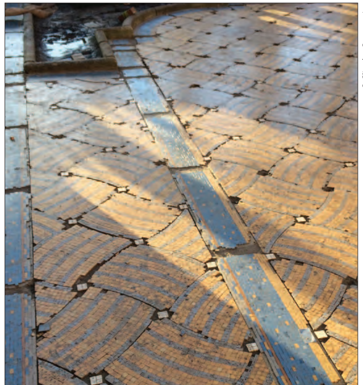
The finished panels being bedded before doing the infilling with joining tesserae
