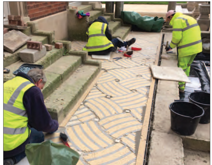
Infilling work on the Upper Terrace, where new tesserae were used
