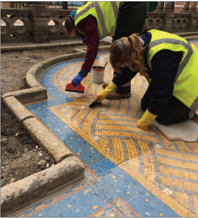
Installed, cleaned and dry, all mosaic surfaces were grouted
