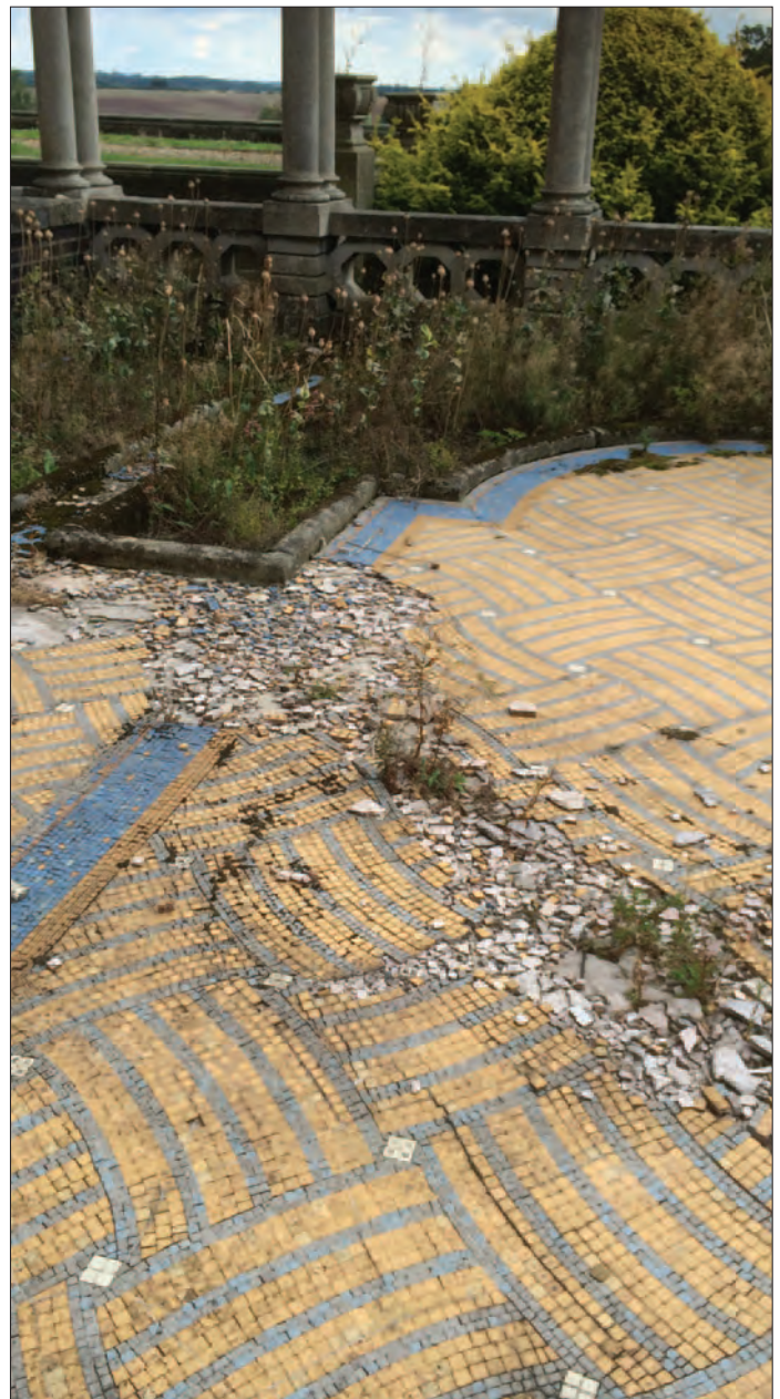
The deterioration of the main floor before conservation work
