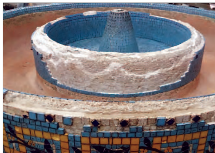
Defective mortar removed and hollow areas re-grouted prior to building up the new core
