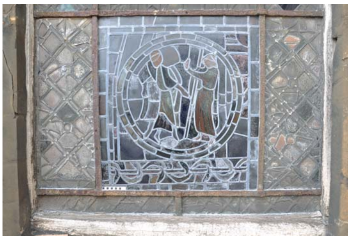
External view of the window with the facsimile panel replacing the broken one
