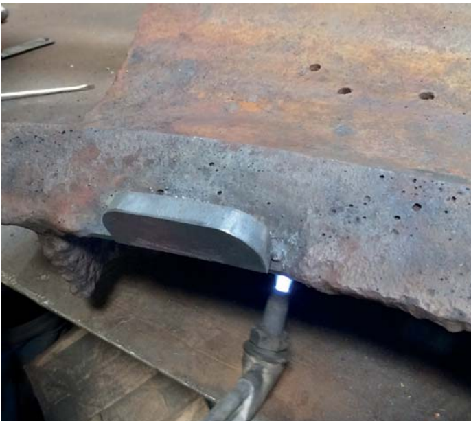
Heat is applied beneath and around the repair
