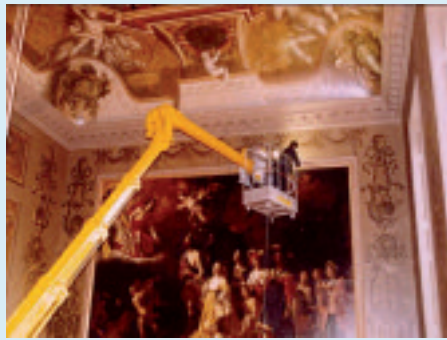
Using MEWPS (Mobile Elevating Work Platform) to access painting at Hampton Court Palace
