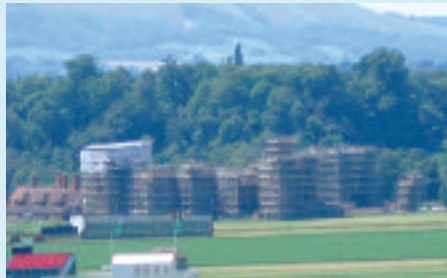
Scaffolding of ruins at Cowdray Park
