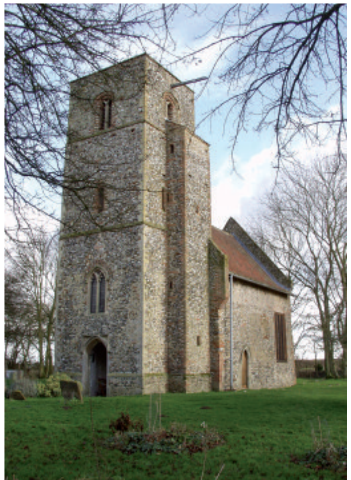
External view of the church from the south west
