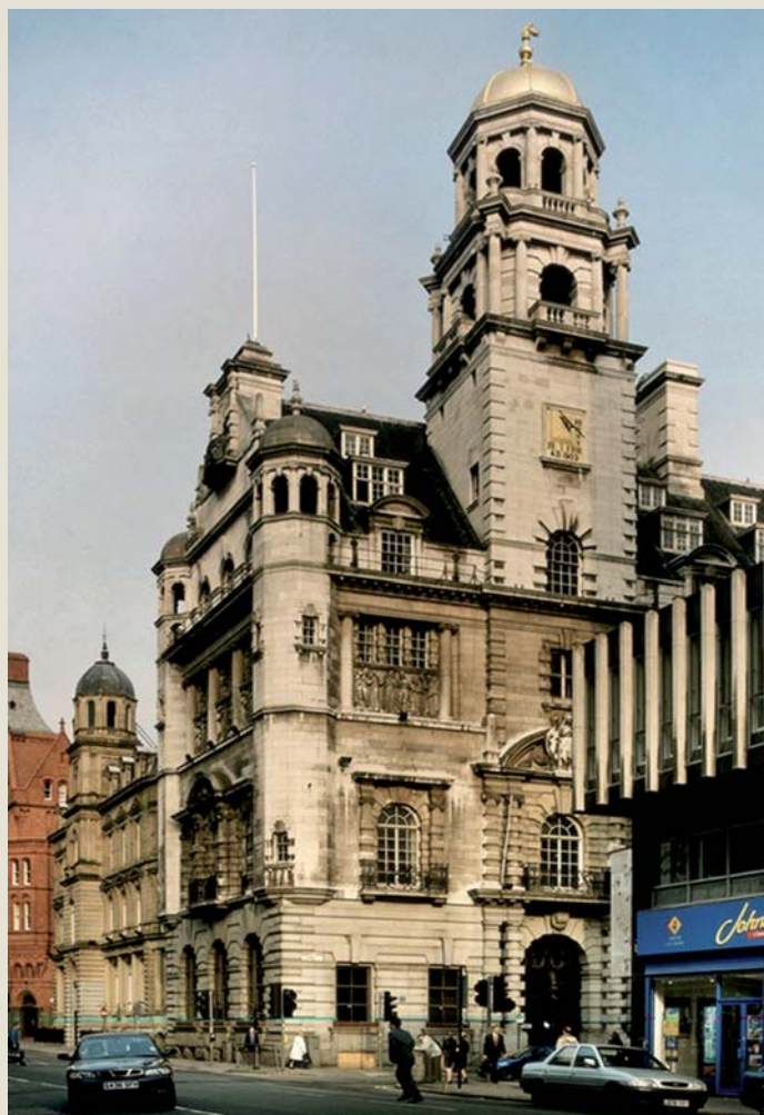
The Royal Insurance Building Liverpool – at risk
