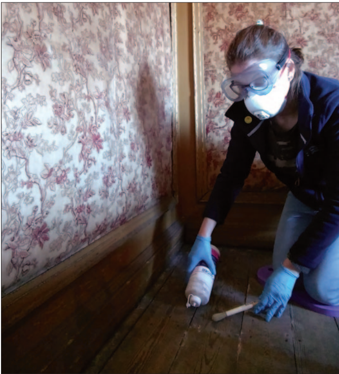
Application of silica dust powder to floorboards
