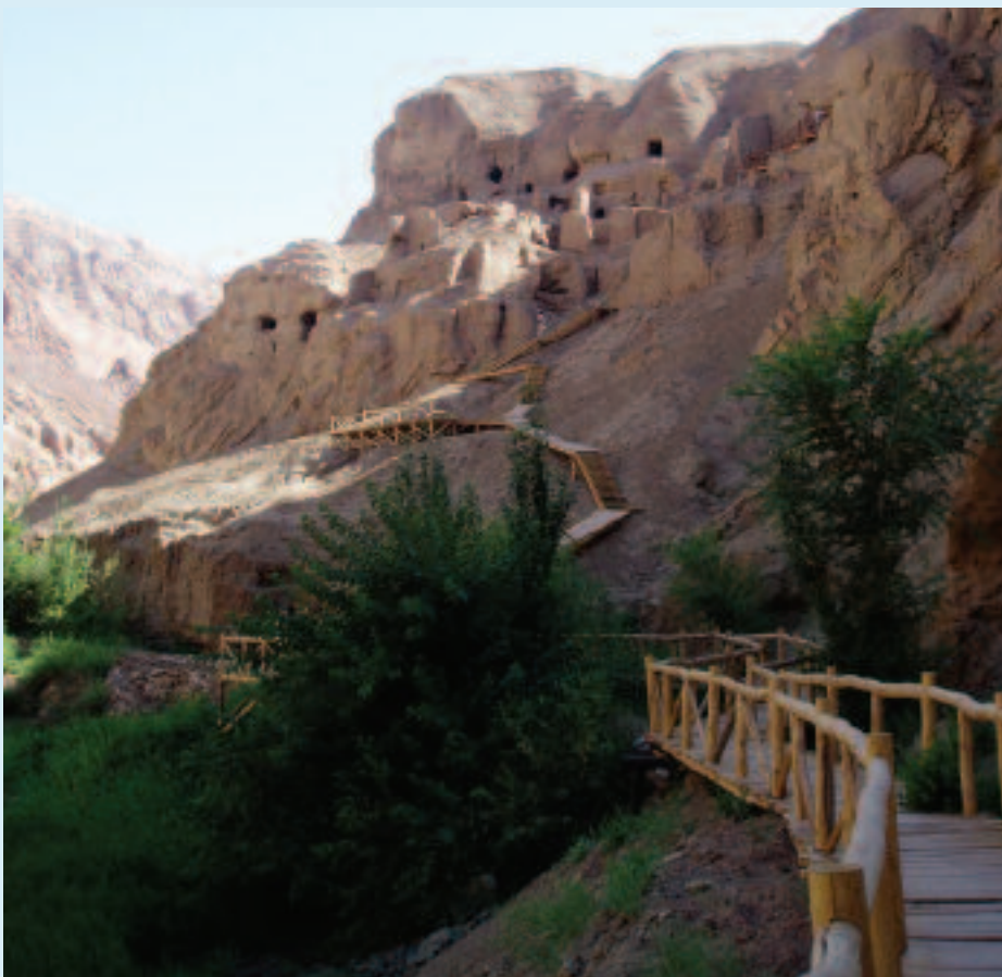
A newly constructed poplar wood walkway gives access to the Tuyuk Grottoes
