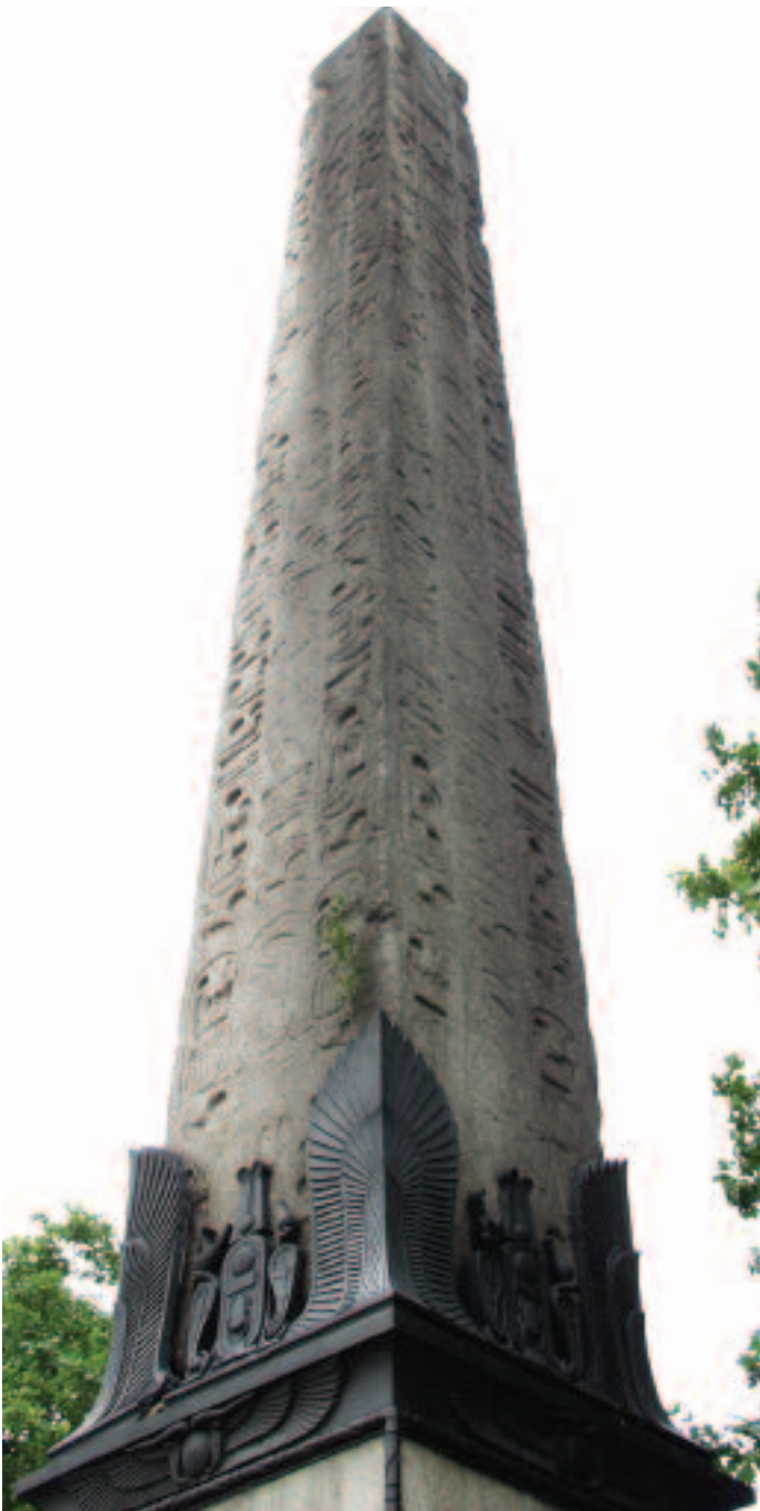
South-east corner, pre conservation
