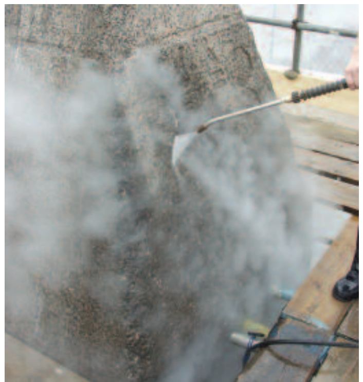
Top level being cleaned with the DOFF system
