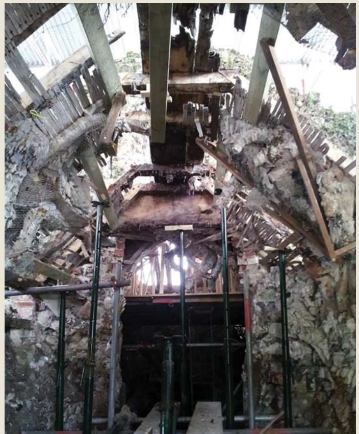
The entrance chamber with the internal supports being installed before the conservation programme can begin
