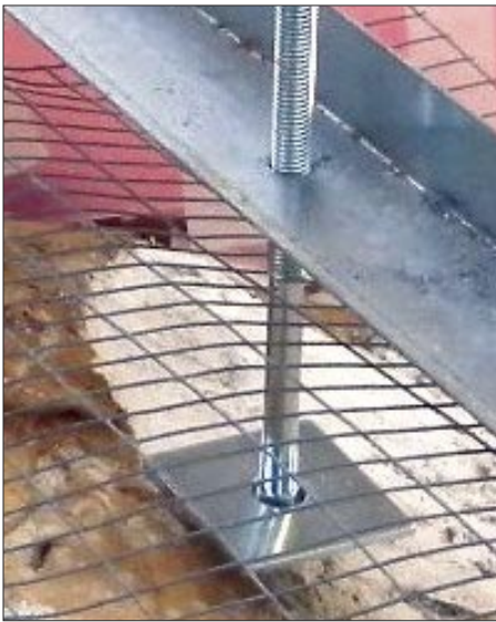
The bolts, weld mesh and plates in position before the resin was applied and the alginate mould of the missing area
