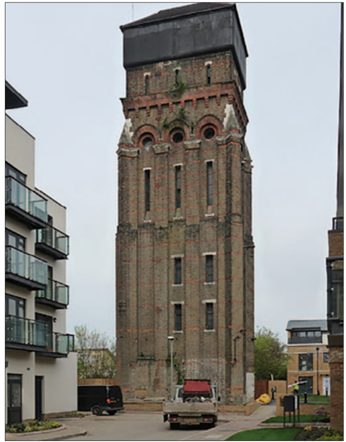
The Lambeth Water Tower before work to change its use
