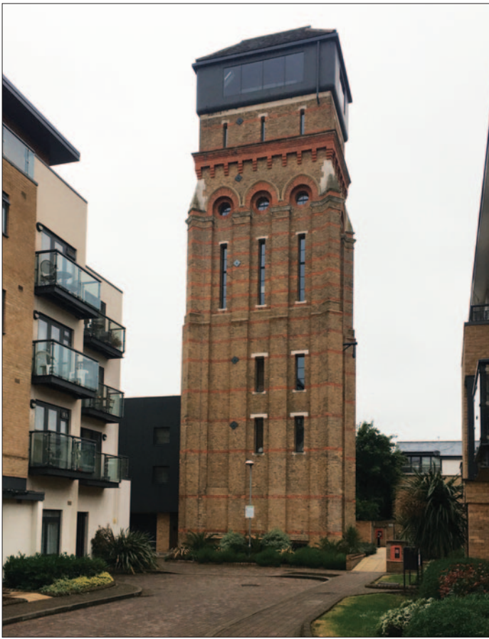
The Lambeth Water Tower after its adaptation to residential use
