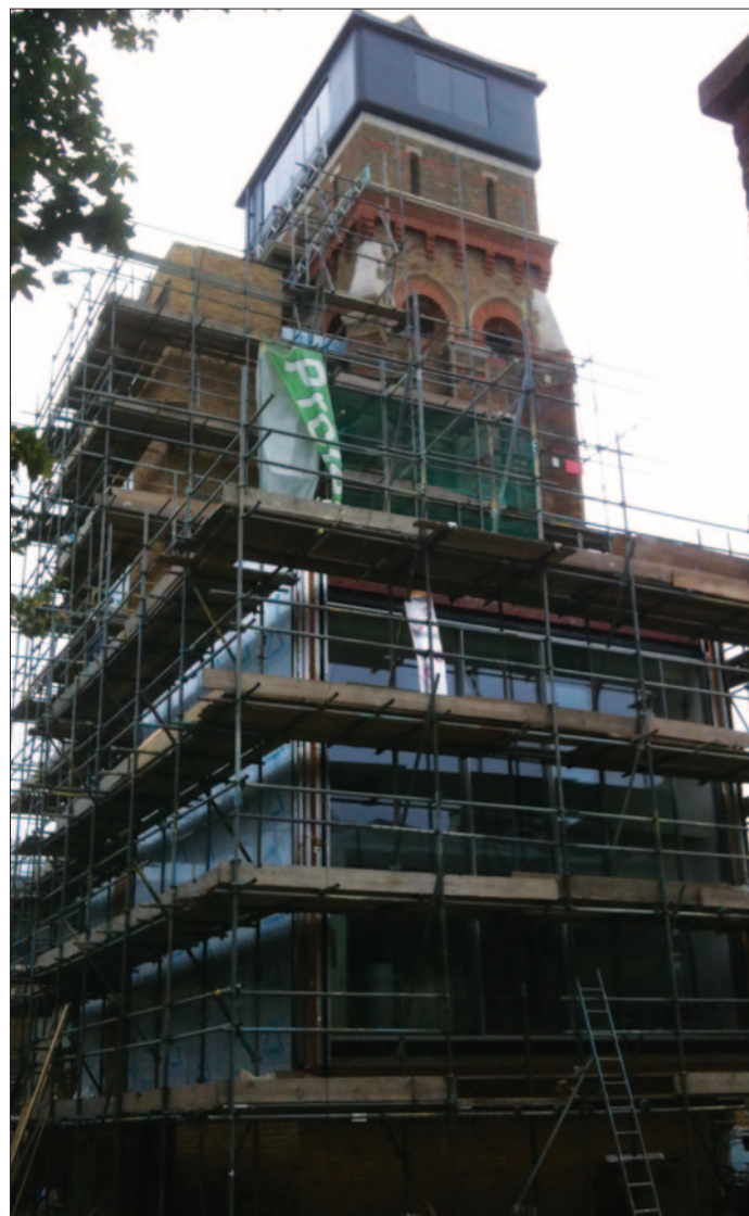
The Water Tower during re-purposing works, 2012
