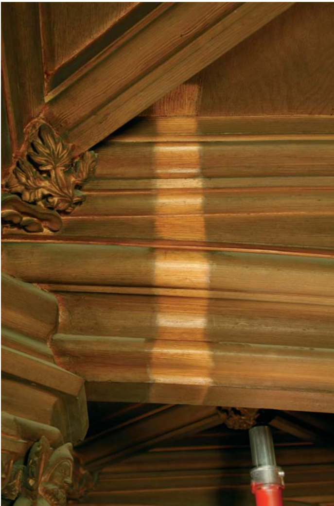
The Library, surface cleaning trial from painted graining on ceiling
