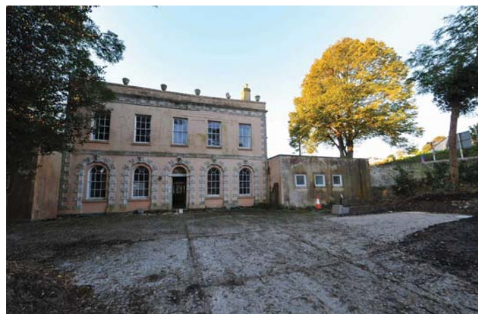
Belmont house in October 2013. Coade stone features liberally embellish its facade
