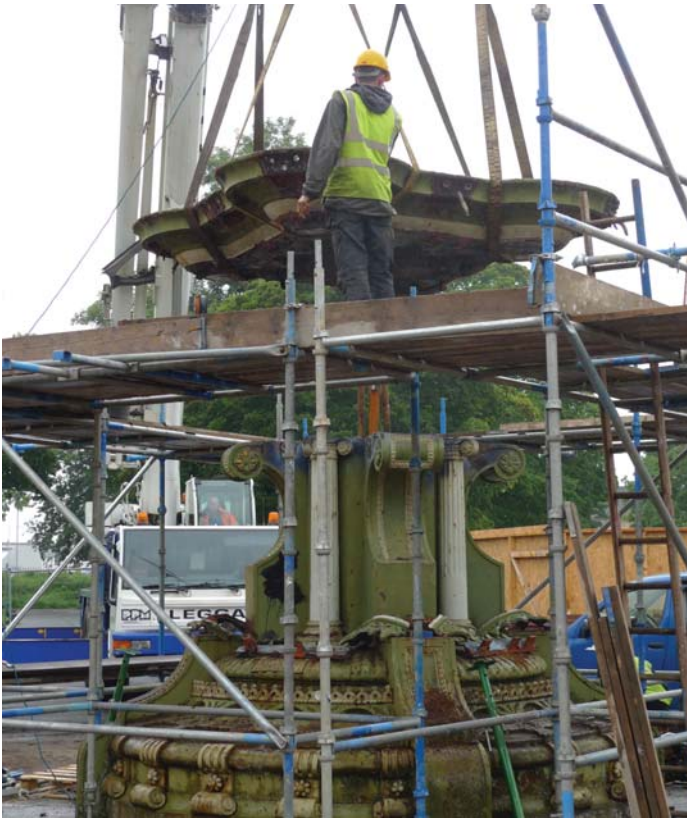
Two tonnes of bowl lifted clear. This is the fourth and final bowl in the cascade, mounted on the buttressed core
