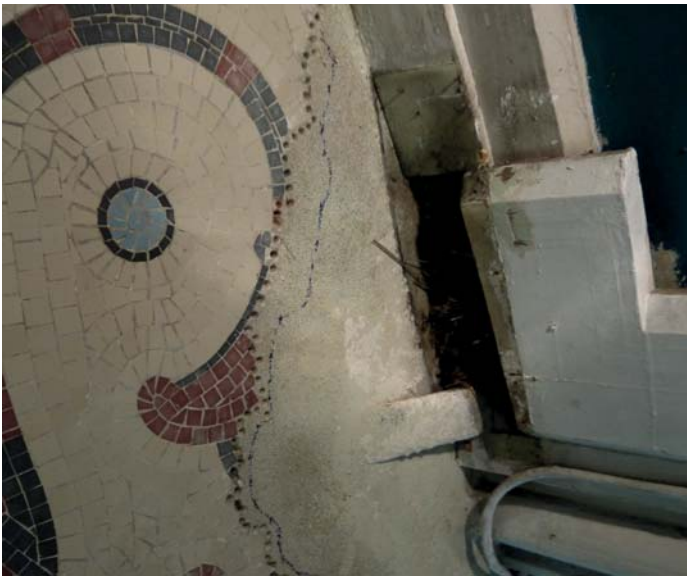
1. The existing rendered surface has been checked for flatness against the surface of the mosaic and high areas identified. These are marked and chain drilled
