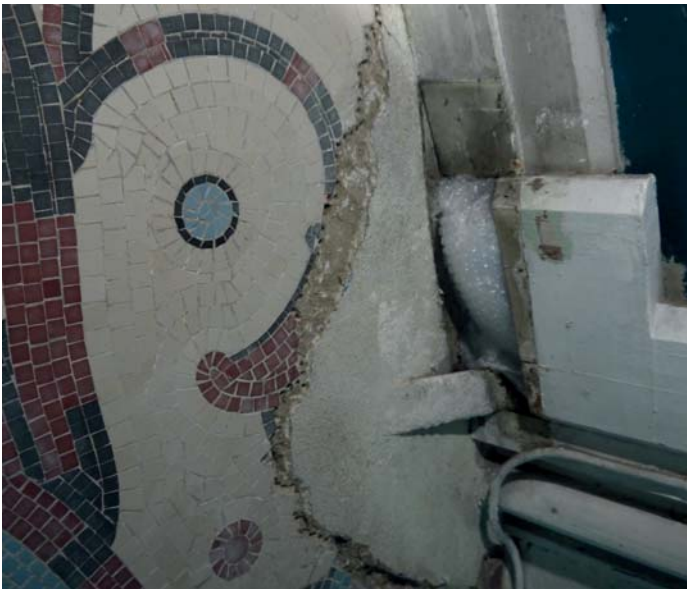
2. The surplus mortar is removed with chisel and mortar
