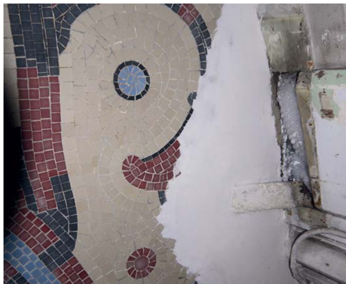
3. New mortar is added and the plaster flushed off square and true to finish
