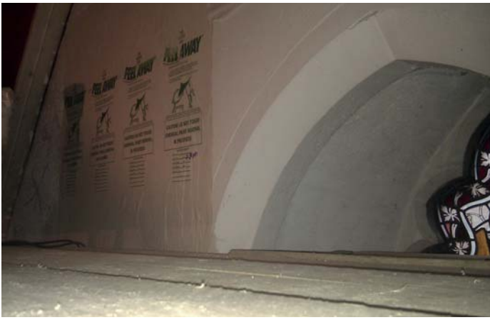
First poultice in place with plastic covering at 3rd lift level
