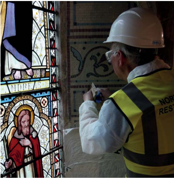
Cleaning the residue from cement grouting and around the stained glass windows on the 2nd lift
