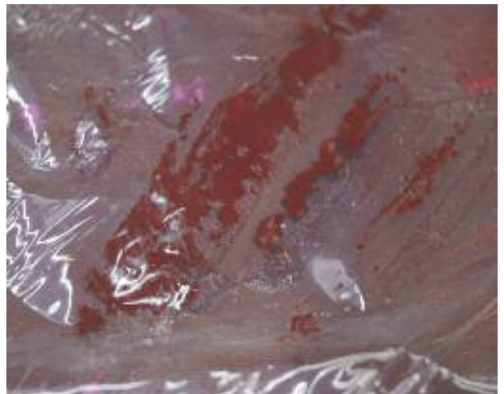
Figure 2: Detail of red paint showing the change in surface texture caused by the polythene.
