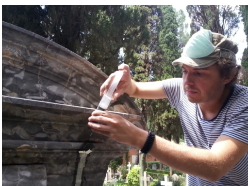
Fig. 1 Injecting the NHL 3.5 grout
