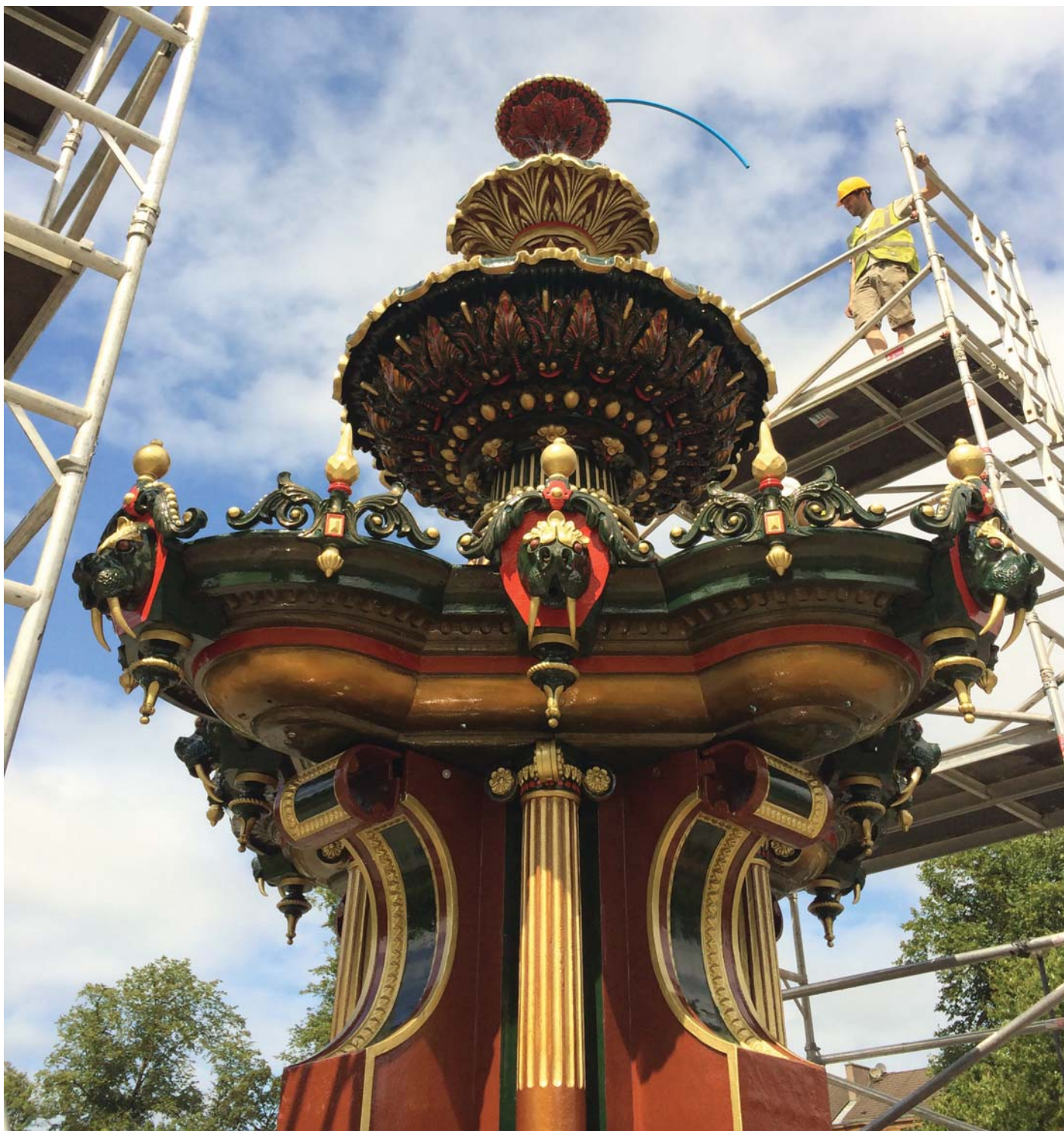
The fountain assembly: all this in a day. The bronzing can be seen beneath the quatrefoil bowl and on the column base
