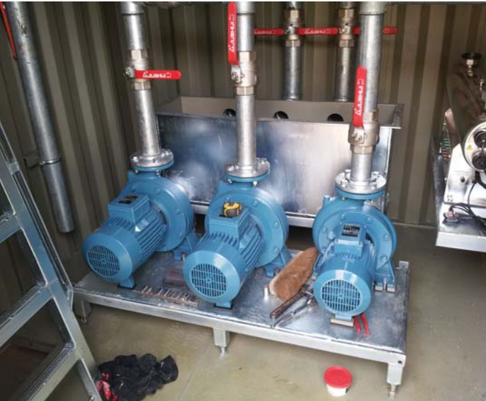
The three powerful pumps with the UV treatment unit and the filter box
