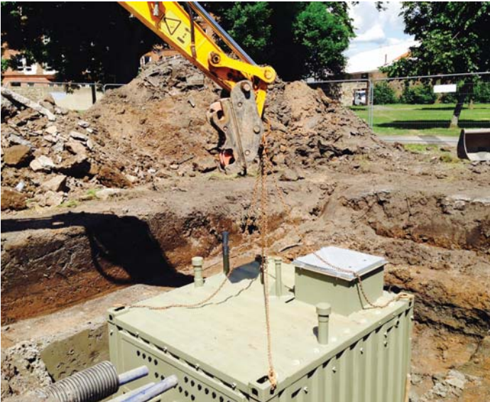
Installing the service chamber
